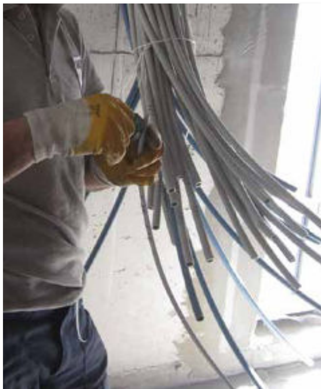
An operator stripping cables during installation.
